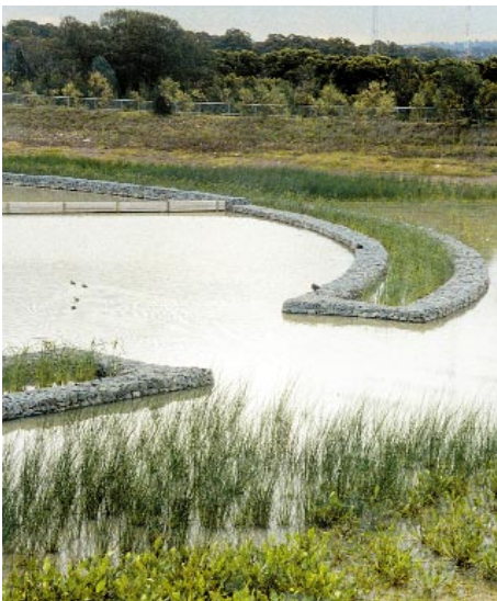
One of the specially constructed ponds, built to treat rainwater from the Olympic site.
